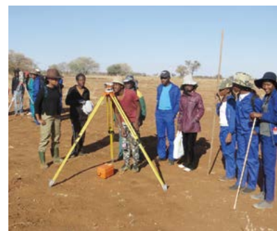
Students of the Namibia University of Science and Technology operate a dumpy level for marking contour lines (Ibo Zimmermann).
