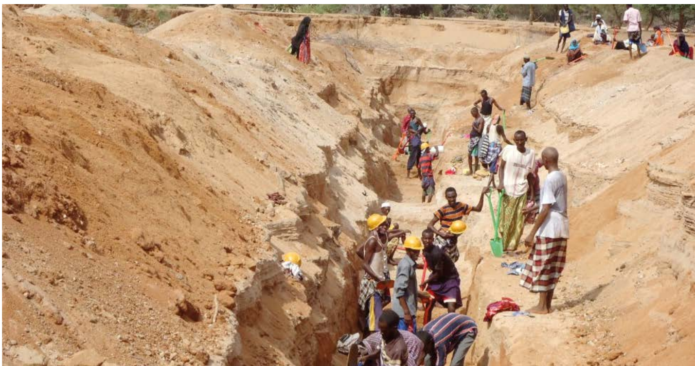
Excavation at Leyhele (IUCN archive).
