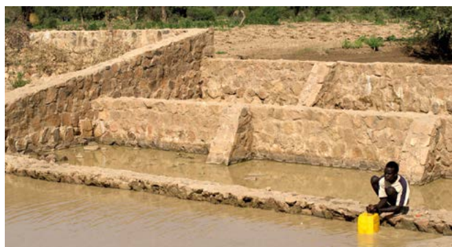
Water-spreading weir, Mali (Klaus Wohlmann).
